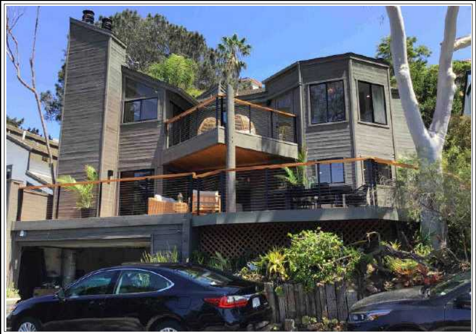
FRONT VIEW OF SUBJECT PROPERTY
